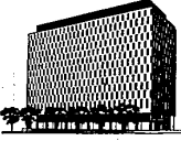
Main Office, Woodward at Ford
