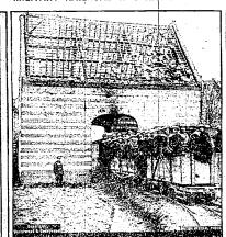
Millinary railroads have the right of way on the western front, s rulned house was not allowed to block this line. The engineers pierced I walls of the house and arched them over, and now the cars filled with te run right through the house on the way to the front lines.
