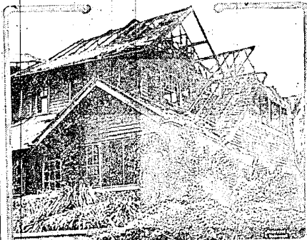
Remains of home of Oscar Lawler, Los Angeles, Cal., which was blown up by a dynamite bomb and filled with two tons of gasolene. Mr. Lawler was assistant United States attorney general for the interior department. Charles H. McGuire was accused of setting the bomb in revenge for the breaking of a will by Attorney Lawler. He committed suicide.
