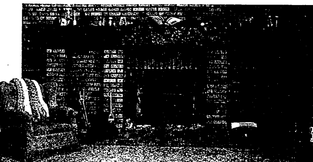
Ernie Rouse's customized heating system utilizes this fireplace that prevents loss of heat common in most other conventional fireplaces. In this system, heat from logs boils water which is used to heat the house.
