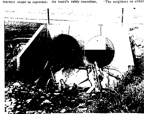
EROSION'S WORK—Erosion has cracked the concrete abutment surrounding the culvert serving the drain running through Lincolnshire Estates. Since this picture was taken, the cracks have widened and the abutment is leaning forward, threatening to fall into the ditch.
