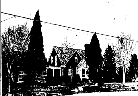
THIS HOME IS CONDEMNED
