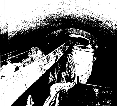
DOWN UNDER — This view is 50 feet down and more than 50 feet into a storm sewer tunnel being dug for the Jeffries Freeway. At the rear a saucer shaped drill face is boring a 10-foot cut. Dirt is being conveyed toward the camera to boxcars behind the photographer. (Observer photo)
