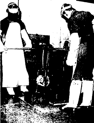
MEN FROM MARS?—Roger Emerson and Charles Schems are the two incognito high schoolers disguised in protective clothing. Students in the machine shop at Farmington High School, they're pouring molten metal, an extremely hazardous occupation. The boys are making usable vites from scrap pieces of raw aluminum. (Evert photo)
