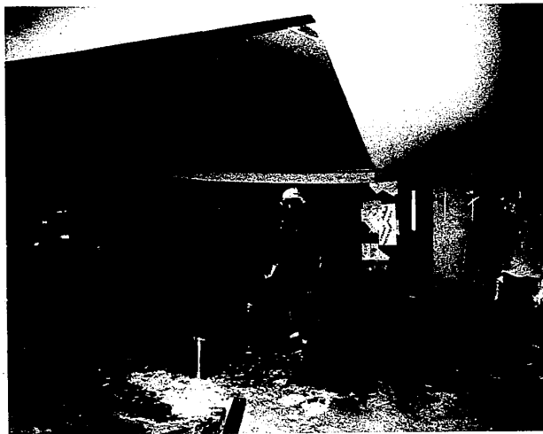
Structural engineers now claim a defective supporting column caused the collapse of the Farmington Hills City Hall roof Feb. 5.
