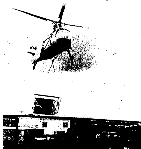
OVER THE TOP -- An air-conditioning unit about the size of an average car is air lifted to the roof of the Topp's Department Store now under construction on Orchard Lake Rd. in Farmington Township. The copter, which can lift up to 5,000 pounds, was used because it's more dependable and quicker than a crane. (Evert photo)
