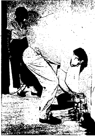
USE EDGER FOR rough sanding of areas not reached by drum sander. Use Coarse discs No. 3 1/2 (20) or No. 4 (16) discs.
