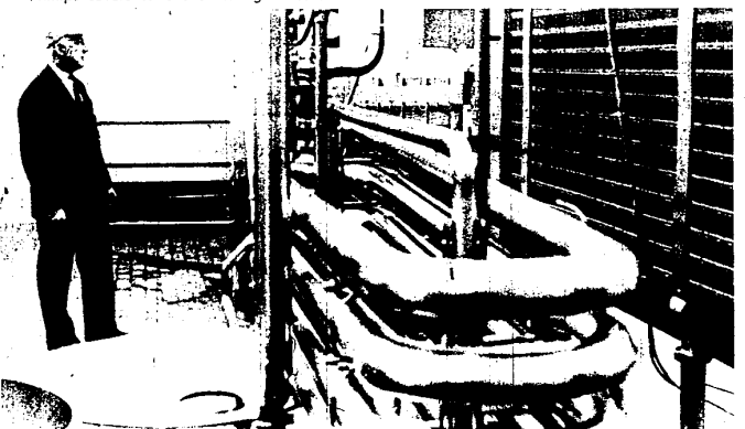
PASTEURIZING COILS — Kroger executive Bob Johnson stands beside the set of coils that holds all milk at 175 degrees Fahrenheit for 16 seconds.
