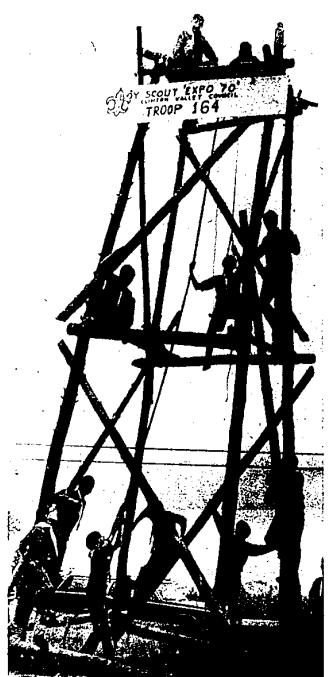
CLEAR VIEW -- Farmington Boy Scouts had a great time climbing the 20-foot signal tower erected near the entrance of the Expo 70 camping area in Walled Lake. The tower was built by locking legs and timber together with rope. (Evert photo)
