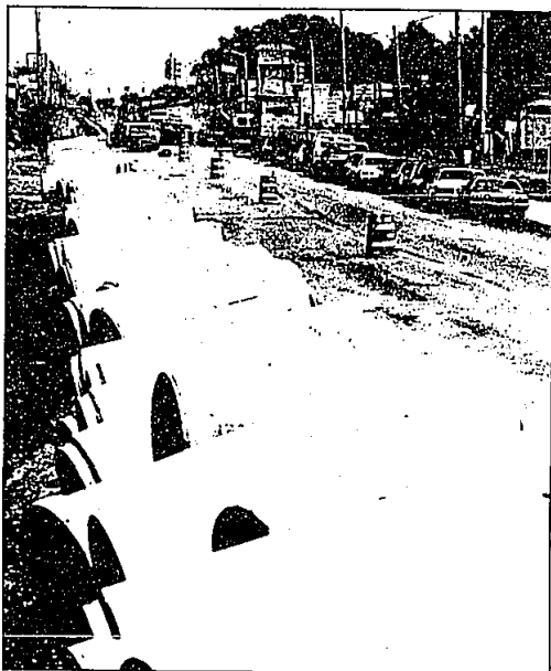
Expansion in Avon Township, Farmington Hills, Troy, Waterford Township and West Bloomfield created most of the work for the drain commission which put in place 400 miles of sewer lines during the peak building years. But with development halted, the drain commission's personnel ranks have been reduced from a peak of 208 in 1979 employees to 59 this year.
