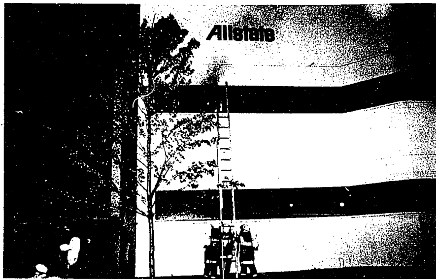
Farmington Hills firefighters battle a blaze at the Bond Street Building, site of the old Bond School, last Tuesday. The fire caused an estimated $75,000 in damages.
