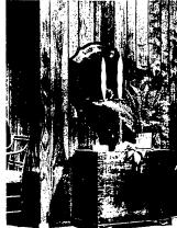
THIS NEW HARDWOOD paneling is enhanced by a different technique in the finish of the wood. Instead of sealer, the stoin is applied to the veneer first, so that the wood takes the stain naturally. This gives the paneling greater depth and life before the pares of the wood are closed with the protective sealer and top coat.
