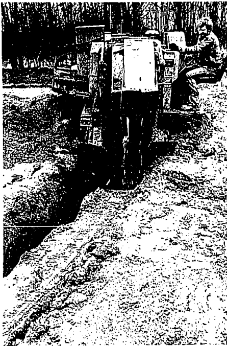
Worker Dan Right uses a Vermeer trencher for the new Crossroads shopping center.
