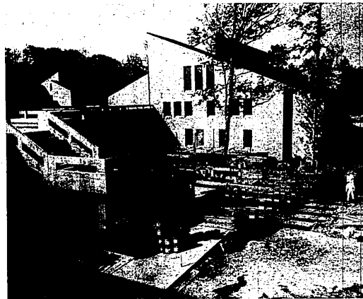
OUTDOOR AMPHITHEATER — A 600-seat amphitheater is being constructed on the Farmington Township campus of Oakland Community College. The outdoor theater will be used for instructional, fine arts programs and for plays, concerts and outdoor speakers.
