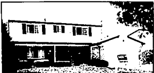
TROY Colonial has good location, updates, 4 bedrooms, 2.5 baths, formal dining, family room with fireplace, Florida room, central air and patio. Finished basement with many possibilities. $139,900. 689-9900 5-A-1441
