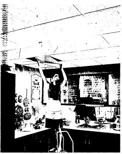
ADAPTABLE for either remodeling or new construction, the suspended ceiling features a combination of incombustible, acoustical lay-in panels and translucent light panels which provide glare-free illumination in work areas. This housewife demonstrates how easily either panel can be
