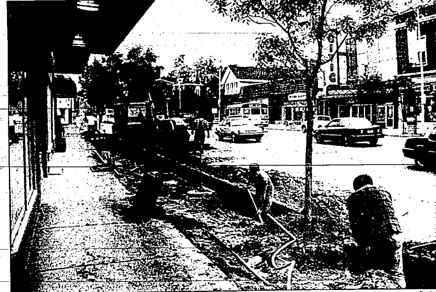
Revitalization is the watchword in downtown Farmington. This photo, taken in 1988, shows workers laying out a grid of wires for new downtown lighting. Farmington, like Rochester, has
