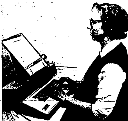
4 Mrs. Nellie Fillmore, a highly skilled puncher, can set type at around five times faster than the old hot type method.
