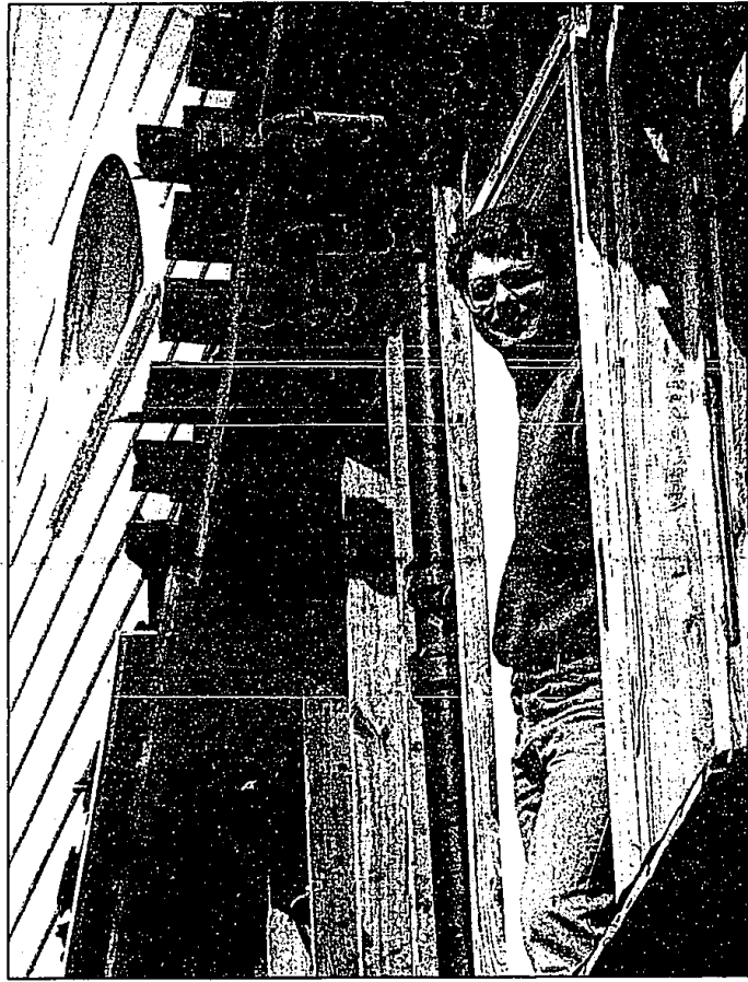
Making ready: Builder Wayne Elliott stands in the doorway of an upstairs bathroom of the historic Kirby White House that is being prepared to be moved a mile south to 10 Mile and Farmington roads.
