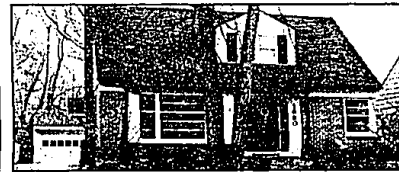
A FAMILY ROOM ADDITION
