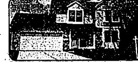
FARMINGTON HILLS. One of the largest premium sites, next to a nature area and a private cul-de-sac setting! Almost new 3 bedroom home with a lovely fieldstone fireplace. French doors to deck. Two and a half baths. Central air. $184,900 626-9100 02-B-8080
