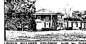
LOVELY PILLARED COLONIAL built by Guldo Grassi on a cul-de-sac site. Library, formal living and dining room, cathedral ceiling great room with easy access to brick walks and bi-level deck. $369,000. (644-6300) B11779
