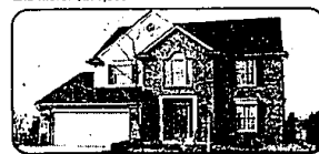
TROY. Prime suburban living in this better than new transferred owners dream home! Loaded with extras. Hardwood floors, upgraded fixtures, impressive family room, master bath with large whirlpool and island kitchen. Beautiful! $238,900 689-8900 05-A-7885
