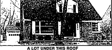
A LOT UNDER THIS ROOF
