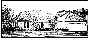
BEAUTIFULLY MAINTAINED Ranch condo set deep in the complex. Open floor plan with soaring ceilings. Lots of wood flooring, recessed lighting, oak kitchen with island and eating area. Atrium, wet bar and greenhouse area. $309,900
