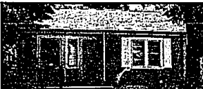
NORTH ROYAL OAK FIXER-UPPER Needs a ton of work! But, you could make a ton of money! Royal Oak price half of average in neighborhood. Perfect for young builder or true handyman. Call listor for details. $42,500
