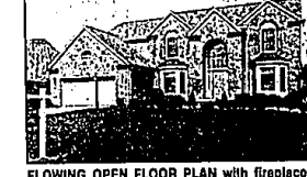
FLOWING OPEN FLOOR PLAN with fireplace between family room and kitchen. Garden corner, bridge overlooking family room, master with gable ceiling. Wood floor in kitchen, den, living and dining rooms. Rochester. $274,000. (651-3500)
