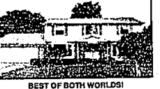
BEST OF BOTH WORLDS! Southfield. Updates galore, meticulously maintained, and over 3,000 sq. ft. 4 bedrooms, 2 full baths, and 3 half baths, family room fireplace, library and attached 2 car garage. $229,000 (OER-20TWY) 810-359-1400
