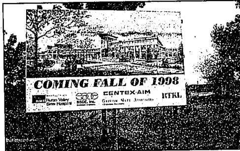
Coming soon: Despite legal arguments over whether area hospital need to expand their operations, some are expanding clinic facilities, such as at Huron Valley Hospital in Commerce Township.
