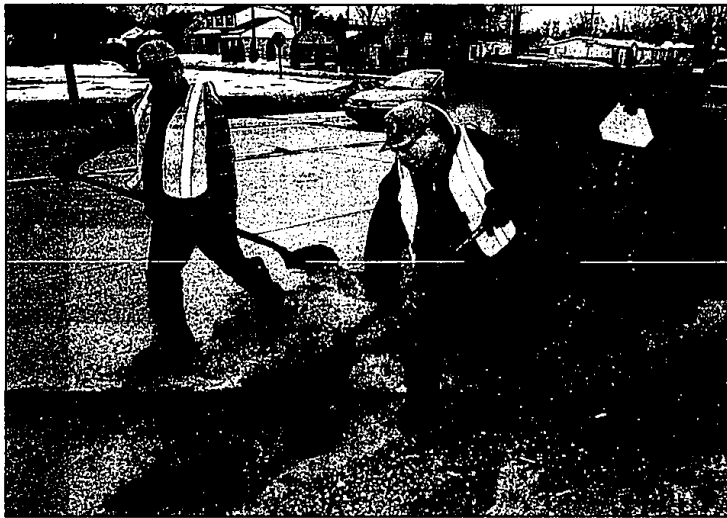
Getting ready: Farmington DPS workers Don Rogers and Don Gould fill Farmington Road potholes with hot patch. Plans for Farmington Road's reconstruction are under way to begin in July.
