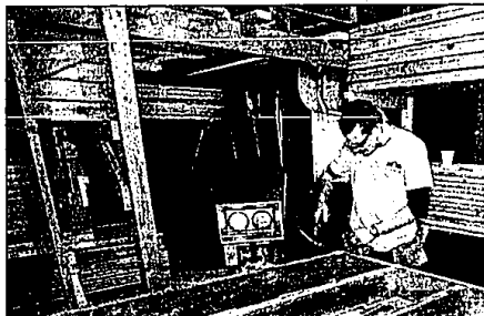
Giving time: Neighborhood Senior Services volunteer Robert Vaclavek of Ann Arbor assembles the framework for a ramp module inside the barn.
