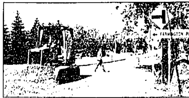
Crews are busy extending the right passing lane on westbound Walnut Lake Road at Farmington Road.
