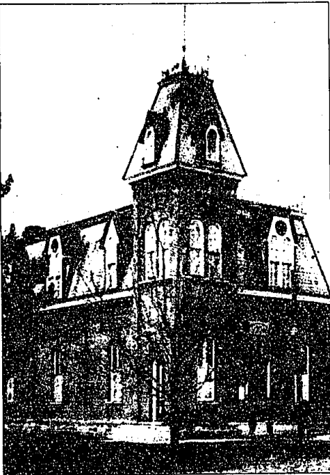
The Township Hall is now the Masonic Hall, site of Lodge gatherings and other community events.
