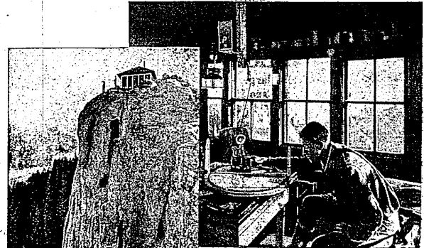
The protection of thousands of square miles of forest land, and the security of lives and property, depend on the alertness of government fire watchers. These photographs show a lookout tower in the Black Hills of South Dakota. Note the range finder and binoculars with which the watcher spots the location of the fire, and the telephons with which he gives the alarm and directs fire wardens to the scene.
