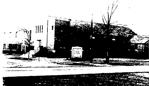
NOW A MODERN church which has been added onto several times. Covenant Community Church serves several hundred persons who come from surrounding areas including Brighton, Allen Park, Livonia, Westland, Southfield and Redford Township. This picture was taken before Beech Daly (street in the foreground) was widened.
