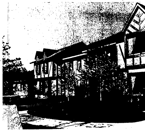
INSTANT STUCCO — A new stucco-like hardboard siding has been developed by Masonite Corporation. Builders and homeowners have found a growing use for it in the half timber construction that characterizes English Tudor and Swiss chalet type exteriors.
