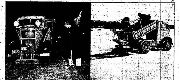
Left: 3,000 individual tests were made during the investigation of winter driving hazards, some of them being conducted at night. Right: Treated abrasives were spread on the frozen lake surface and demonstrations made of their effectiveness in skidproofing. Photos courtesy National Safety Council
