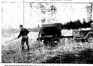
ns have seen this odd looking machin work because it is "custom built thers of the Michigan department of to must invent as well as build the ctured is the "booster" unit which an who hast the "booster" unit which smothers grass and forest-hoor fires with a loglike spray produced at 250 pounds pressure. Twenty of these are now
