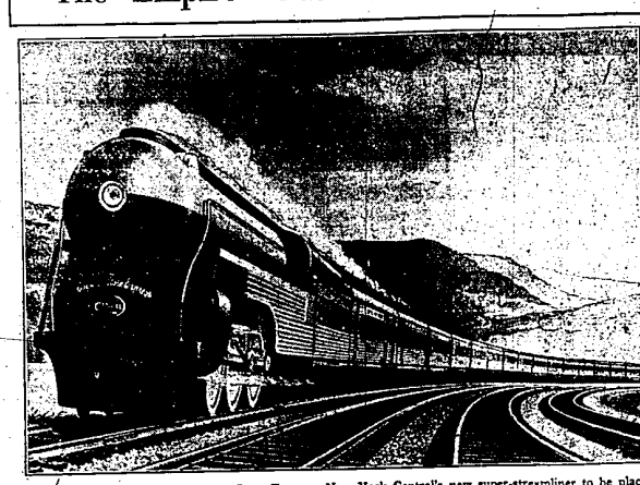
FIRST picture of the new Empire State Express, New York Central's new super-streamliner to be placed in service within a few weeks between New York, Buffalo, Cleveland and Detroit. Its 32 stainless steel cars are now nearing completion in the Philadelphia shops of the Edward G. Budd Manufacturing Company, while its streamlined locomotives will soon be completed by the New York Central's shops. Hailed as the world's most modern day train, it will be operated each day in two sections of 13 to 16 cars each.
