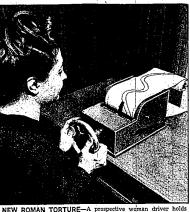
NEW ROMAN TORTURE—A prospective woman driver holds a wheel which regulates a pencil traveling across a twisting "paper road," at Rome's Institute of Technical Psychology. The test is designed to show the aptitude and speed of adjustment of drivers w the aptitude and speed of adj and is given free by the institut
