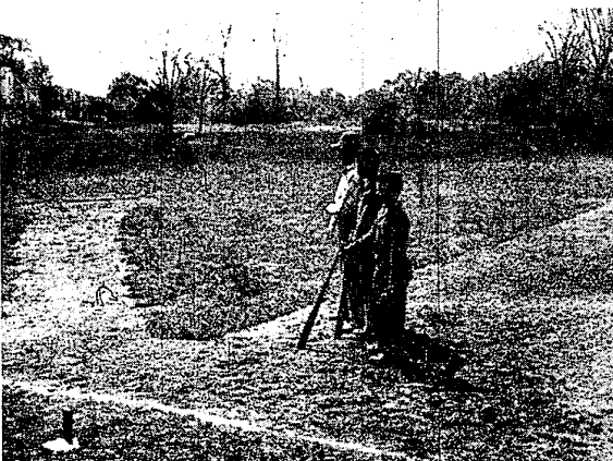
IT WON'T BE LONG NOW... It is probably that these young ball players are saying as they gaze over the "Little League" baseball diamond now under construction in the City Park.
