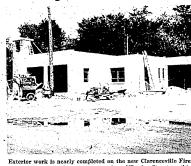
Exterior work is nearly completed on the new Clarenceville Fire Hall building now being constructed on Wheeler Street as this photo testifies. The street rower in the left hand corner of the picture is being finished up and the roof is being poured. The building is expected to be completed in time for the November 4 Presidential Election. Voters of Precinct Two of the township will cast their ballots at the booth located in the new building
