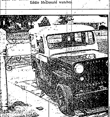
LOOK, NO WALKING—This mailman doesn't have to walk a step on his suburban route in Toledo, Ohio. That's because he's got the first American car in 30 years that features right-hand steering. The Jeep, specially built for the Post Office Department, enables the carrier to drop mail into letter boxes without leaving his seat. When put into widespread use, this design promises to save the department much time and money.
