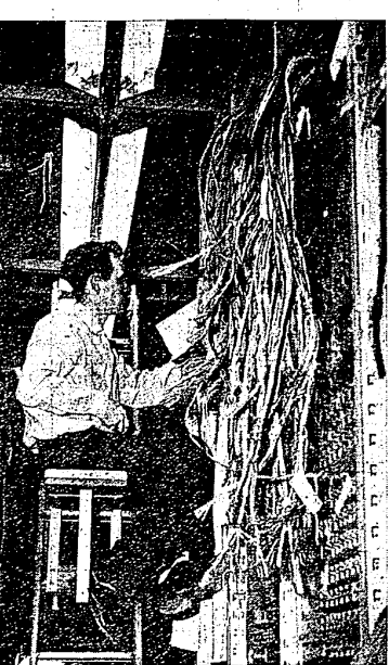
SLIGHTLY CONFUSED is Frank Kayfer, of the Western Electric Company. He is faced with the tricky task of separating multi-wired cables into individual circuits which will permit intricate switching equipment in Farmington's new dial telephone office.
