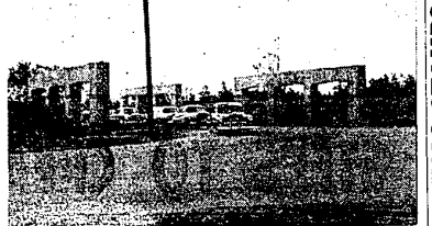
CONSTRUCTION work on the piers which will support the bridge over Farmington Road for the new Farmington to Brighton Expressway have now been completed. Work has been started on back-filling from the piers on an incline for the road. Contracts will be let October 19 for the construction of two additional bridges for the project. One will carry traffic on Ten Mile Road over the Expressway and the other will provide an overpass for Novi Road.
