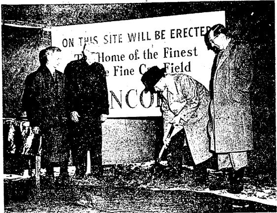
NOVI TOWNSHIP officials looked on happily last Friday as the first shovel full of dirt was turned at the site where the new Ford Motor Company Lincoln automobile plant will be constructed on Wixom Road a half mile north of Grand River. Turning the first shovel of dirt is Gen. D. Mills, a Ford vice president and general manager of the Lincoln Division. Township officials looking on, left to right, are: Earl Stankin, clerk; Frank Clark, trustee; and Ezra Blanton, supervisor.
