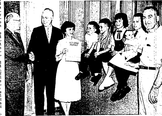
A BUILDING MILESTONE was reached by Farmington Township this Tuesday as the 10,000th building permit was issued by the Township Building Department. Pictured above congratulating the family that will reside in the home scheduled to go under construction soon in Canterbury Commons is
